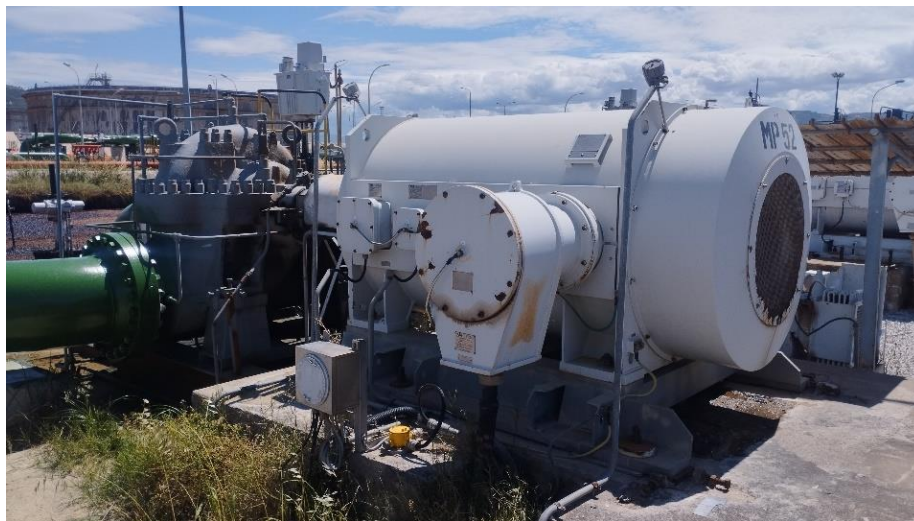
Figure I-7 : Motopompe de condensat
