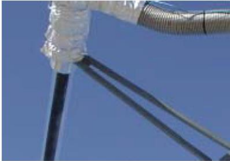
Figure 2. 5: le support de tube absorbeur [76]
