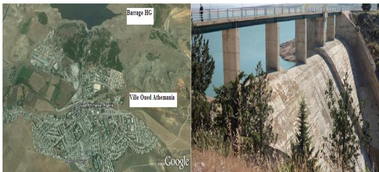
Figure 1-6 : Barrage Hammam Grouz
