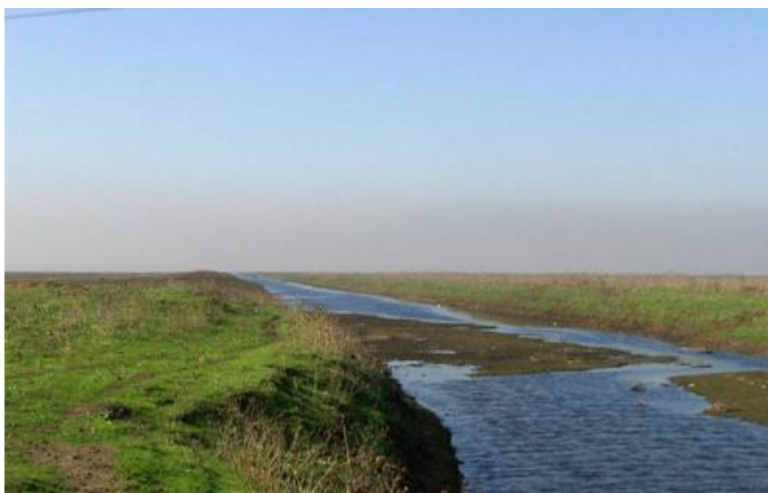
Figure 10. Canal principal (GHI, 2009).
