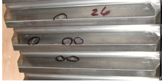
FIGURE 1.2 – Pitting ou piqûres "Engrenages"
