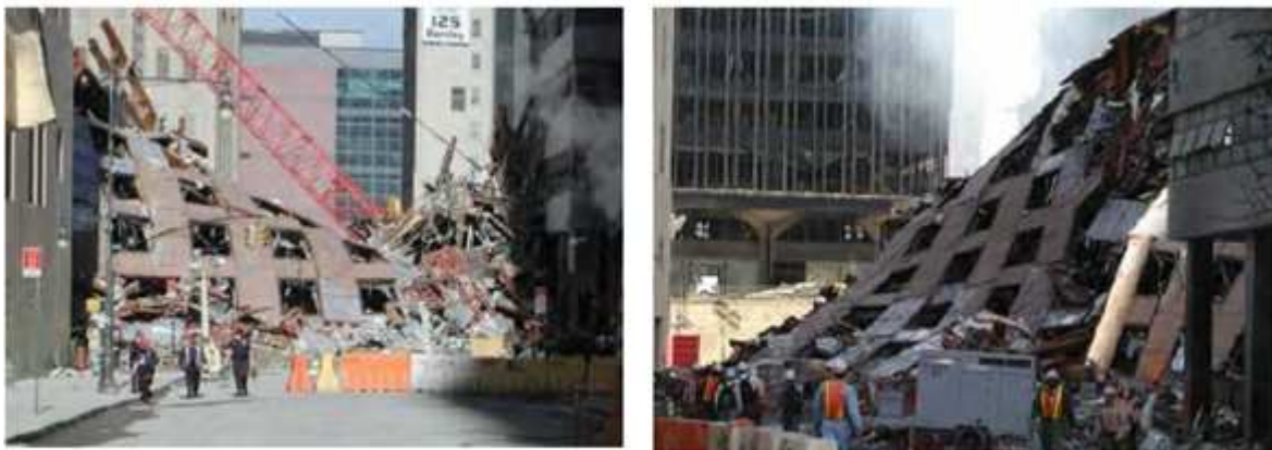
The World Trade Center Building 7 after the collapse due to fire [23]
