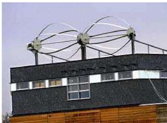
Figure 1.4 : Eolienne de type Darrieus (Wind Wall) [17]
