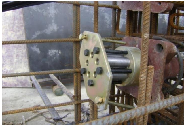
Figure 11. Anchorage plate (passive anchorage).
