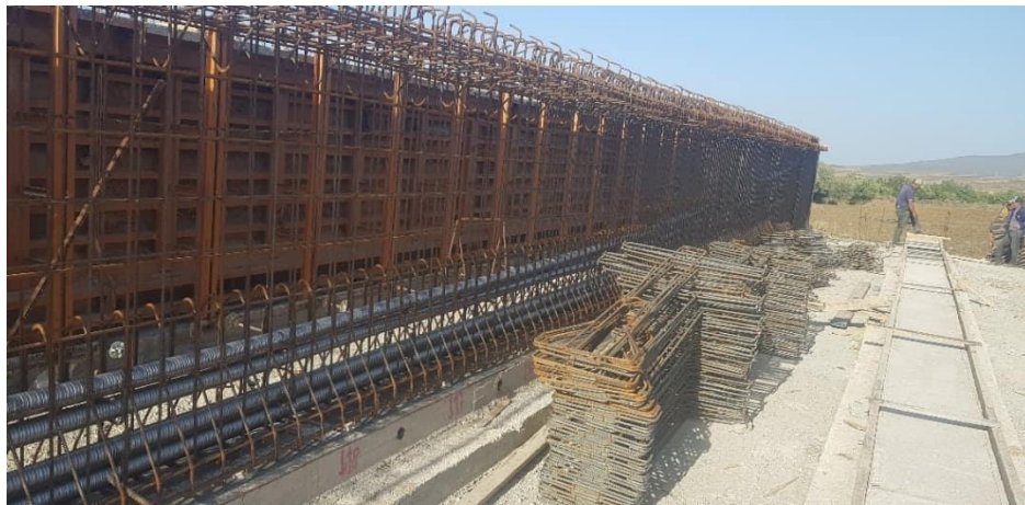
Figure 02. Placement of ducts in the formwork.
