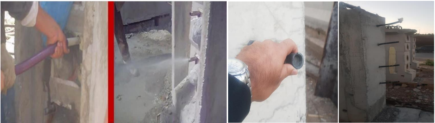
Figure 05. Filling the ducts with injection grout.
