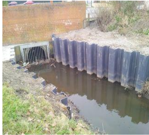
Fig II.6. Sheet pile walls made of metal profiles.
