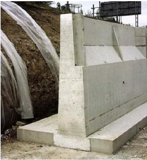
Fig II.3. Reinforced Concrete Cantilever Wall.
