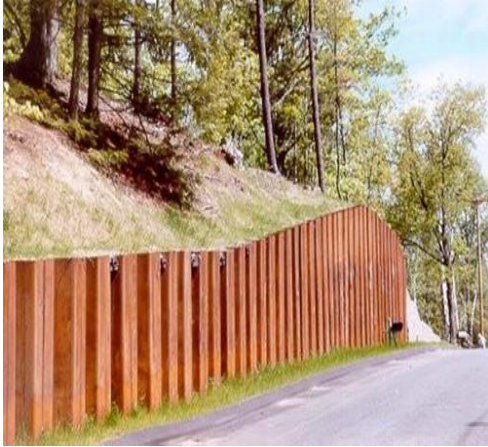
Fig II.6. Sheet pile walls made of metal profiles.
