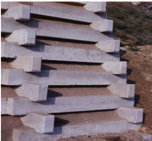
Fig II.5. Gravity wall with precast elements.
