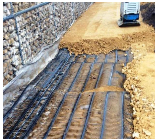
Fig II.8. Earth structures reinforced with geotextiles.
