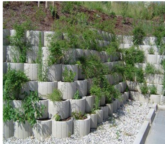
Fig II.5. Gravity wall with precast elements.
