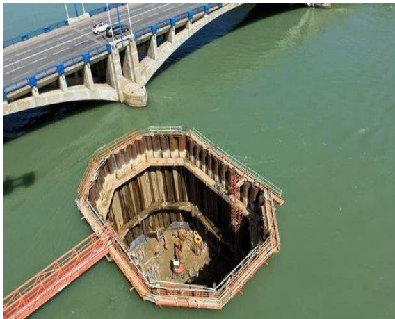
Fig II.7. Cofferdams for the construction of a bridge pier.
