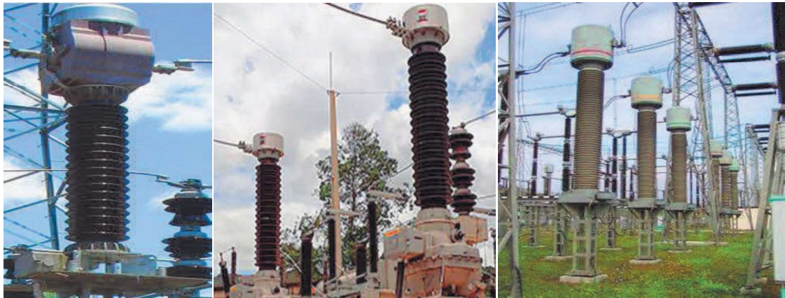
Fig.5.10 Voltage transformer
