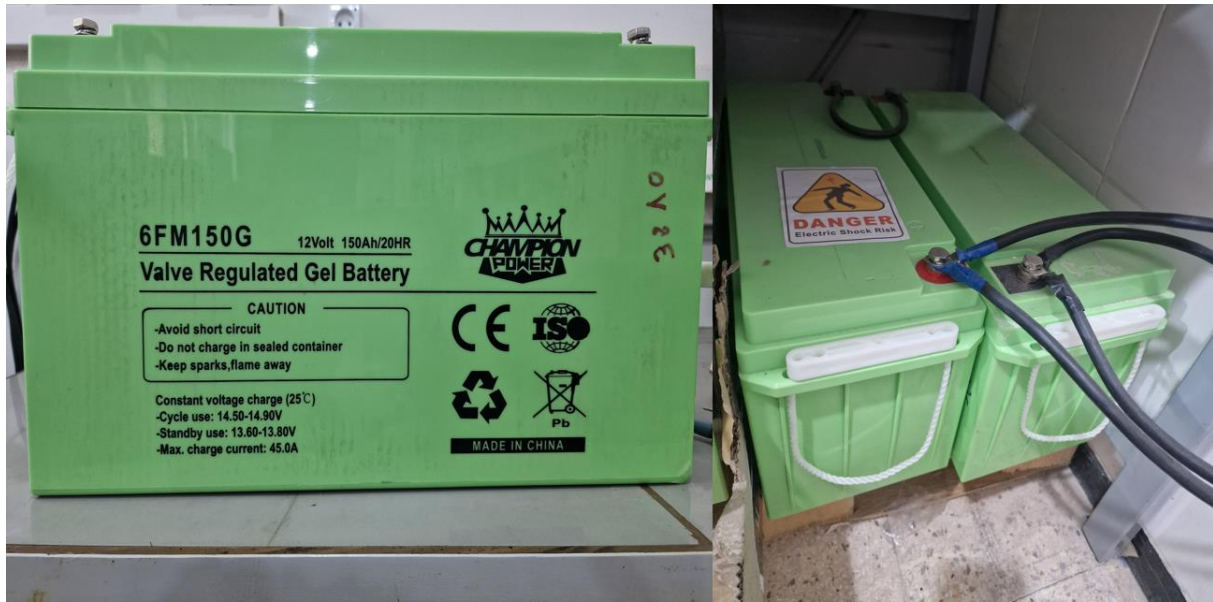
Figure 4.2.3.3 Battery Specs and Connections
