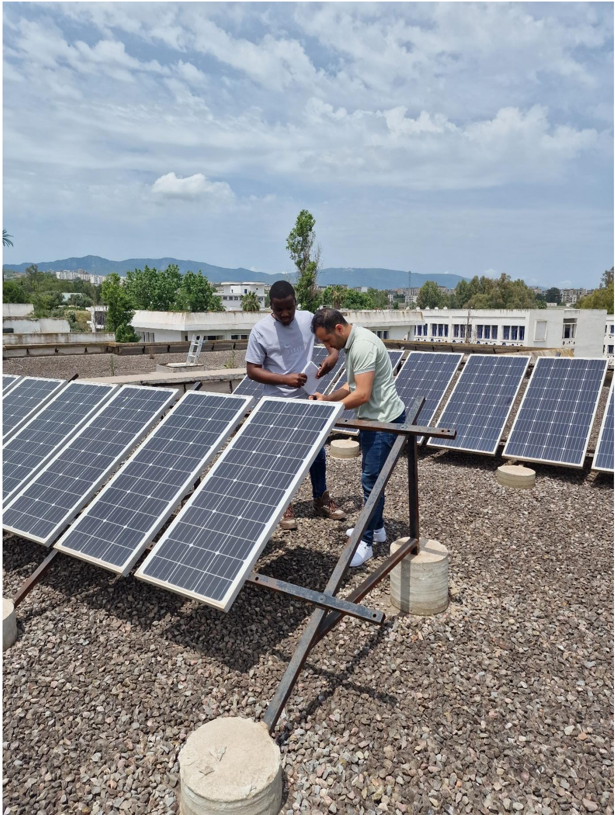
Figure 4.2.2 Modules installation
