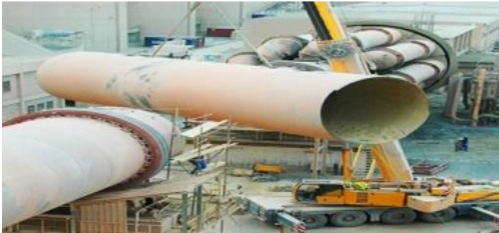
Figure III.5 : Virole de four cimenterie.
