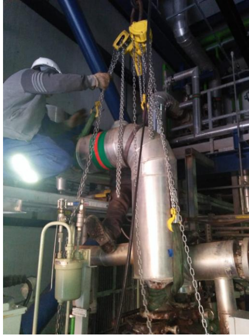
Fig IV.5.Pipeline Unclamping.
