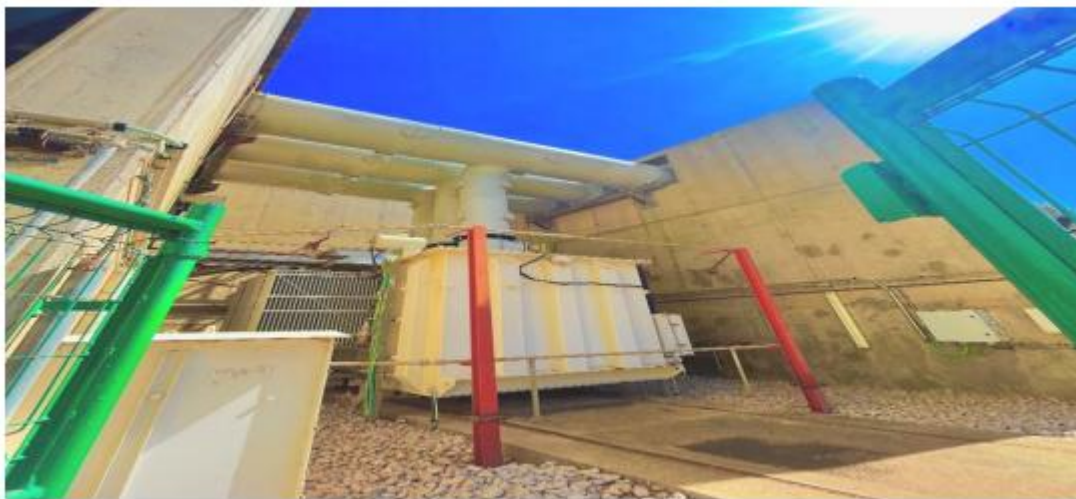
Fig I.16. View of the extraction transformer.
