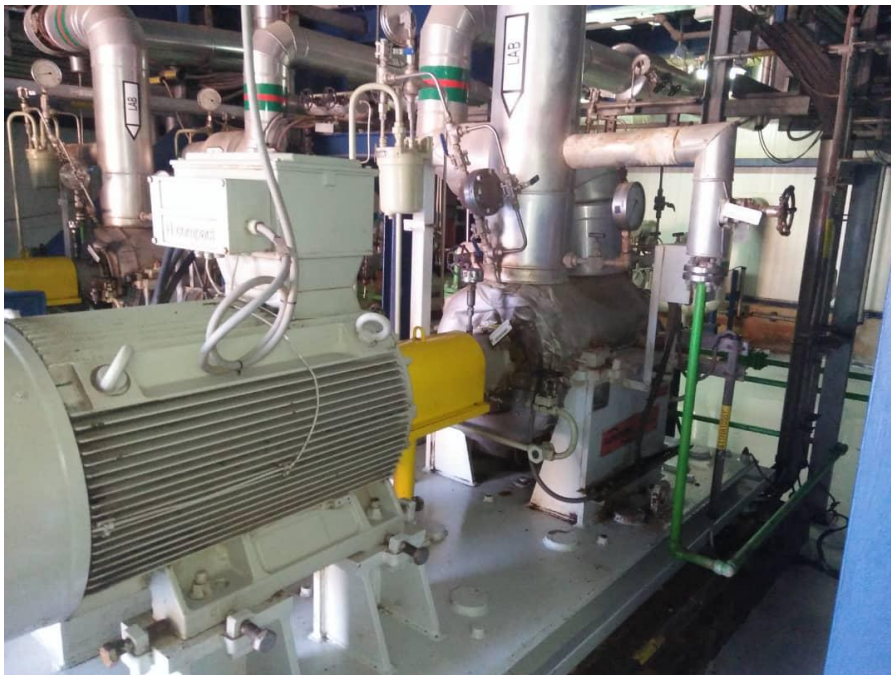
Fig I.19.(MP) Feed Pumps.
