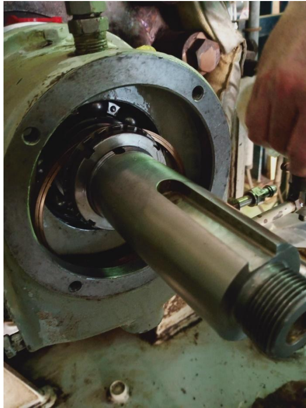
Fig IV.7. Pump motor uncoupling and coupling cleaning.
