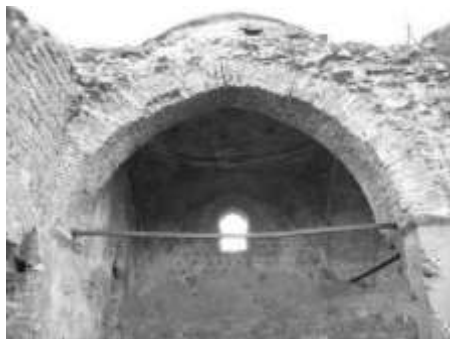
Figure I 22. tie bars made of iron tension members
