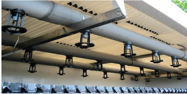
Figure III.5: Rampe de dispersion
