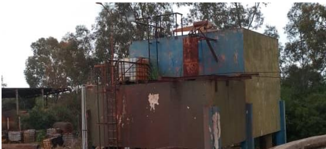
Figure II.01. Le brise charge.
