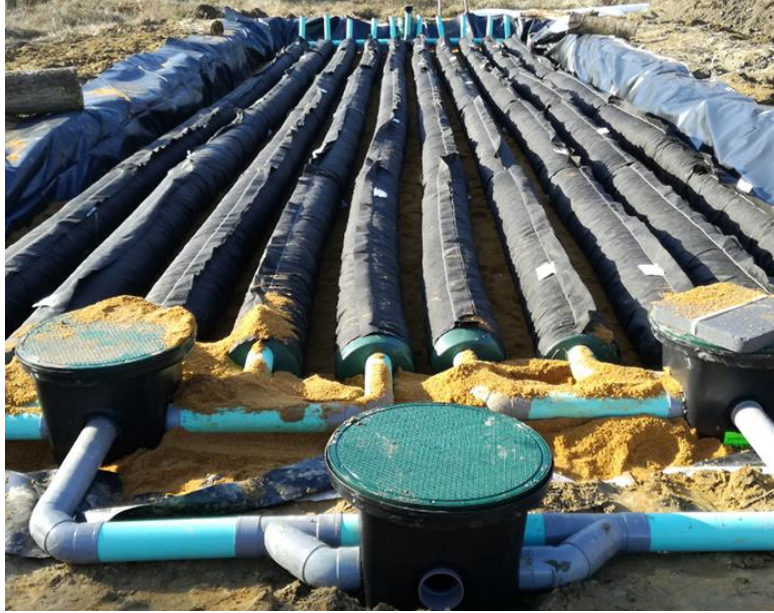
Figure 17 The semi-final installation of the enviro-septic
