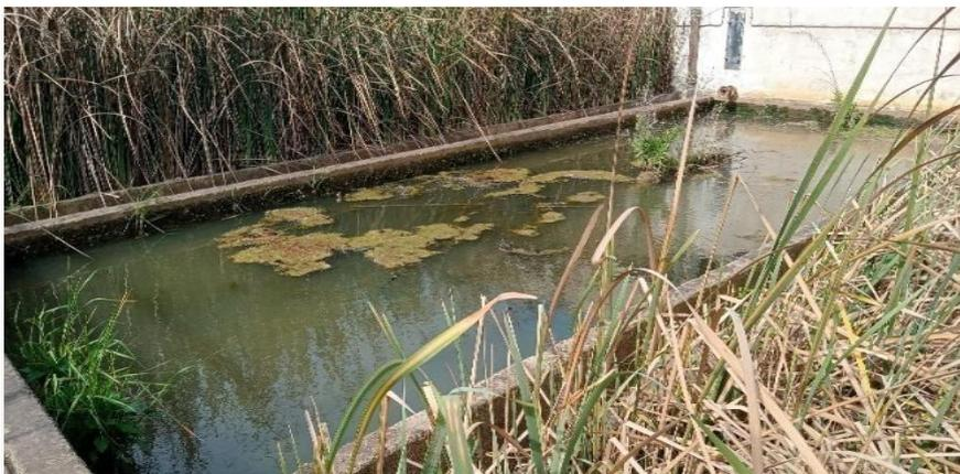
**Figure I.14 :** La filtration a sable.
