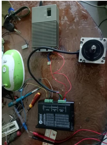
Figure 32 : wiring the high voltage section
