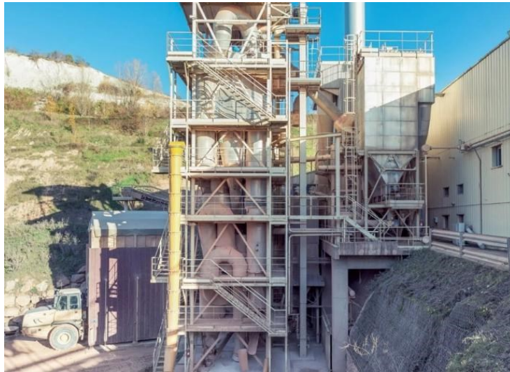
Figure I.26. Four de calcination
