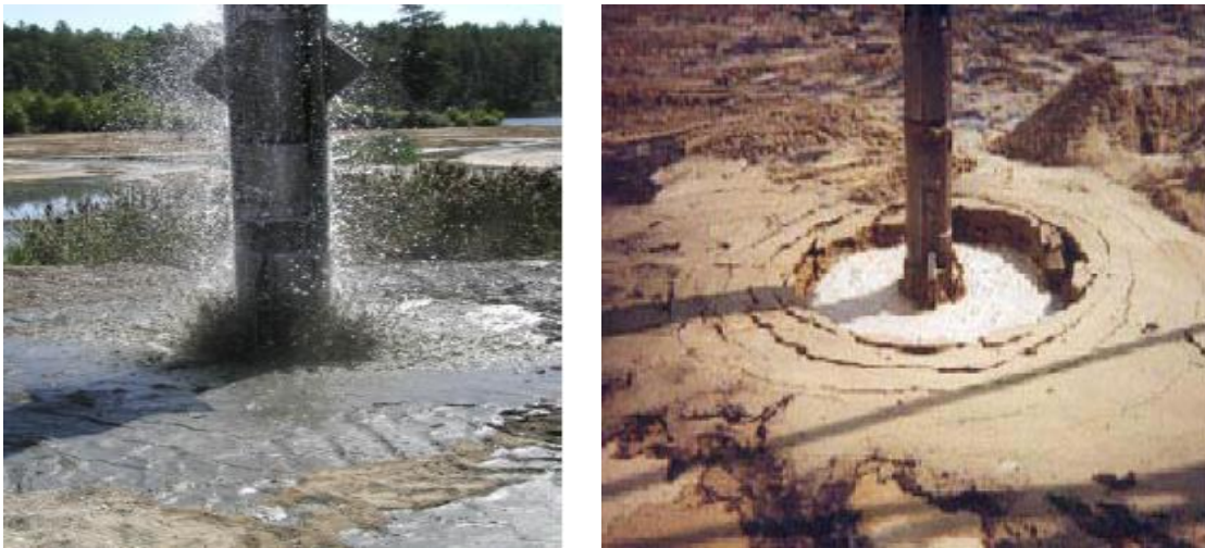
Figure II.19. Liquéfaction du sol
