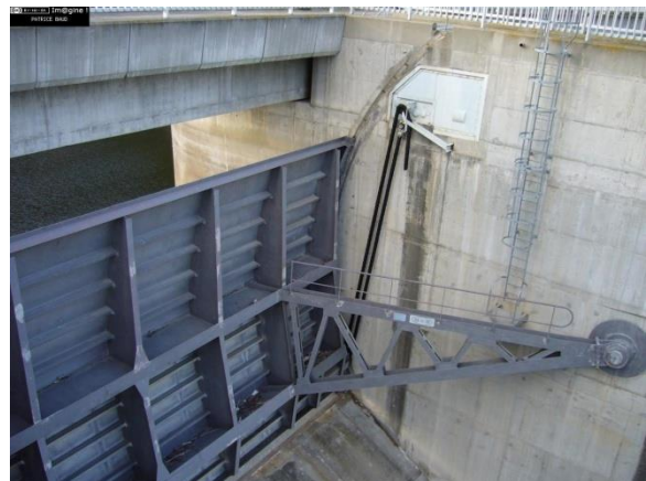
Figure 58 : Vanne segment (Delliou, 2003)
