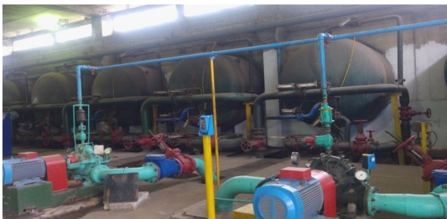
Figure I.5: Salle des pompes.
