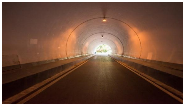
Fig. :1.8 Tunnel routier
