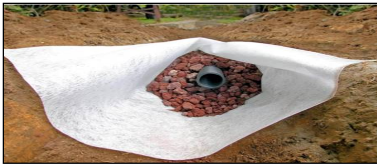
Figure 1.29 Drainage de surface
