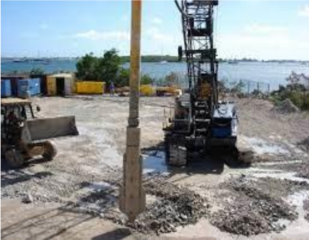
Figure 1.7 : Vibro-compactage.
