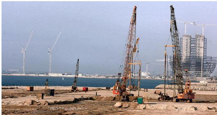
**Figure 1.11**. Vibrocompactage.
