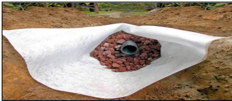
Figure 1.29 Drainage de surface
