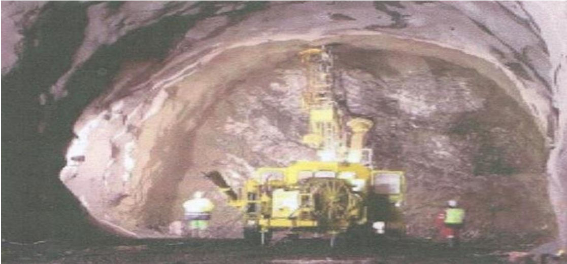
Figure I.8 : Creusement a plain section.
