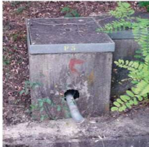
Figure 18 : Drainage profond
