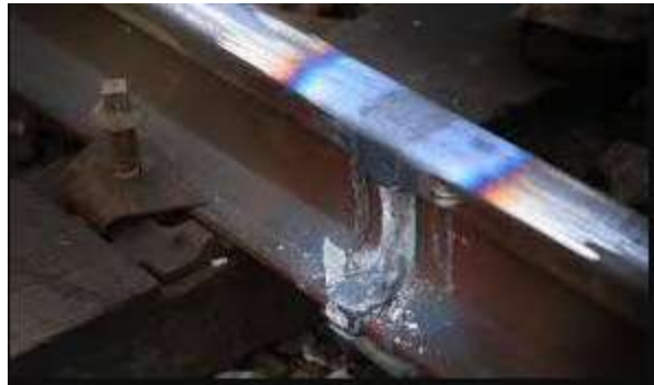
Figure II.18: Soudure aluminothermique (la finition)
