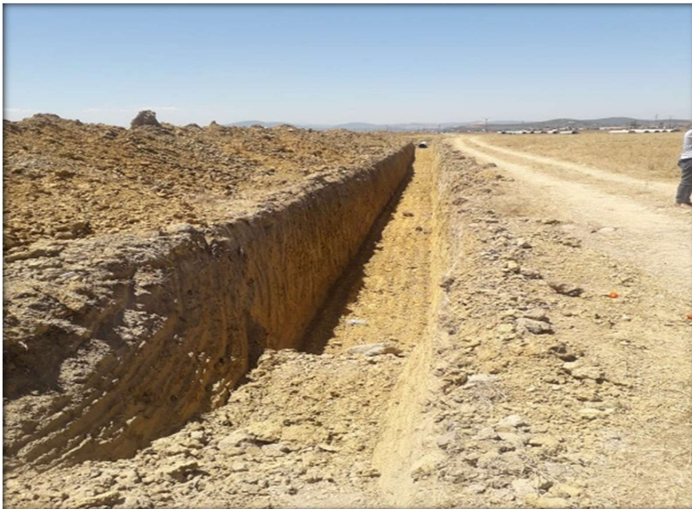
Figure 39-Tranché de la pose
