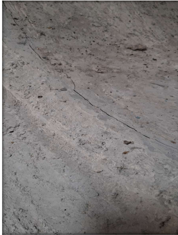
Figure 45-fissures transversal
