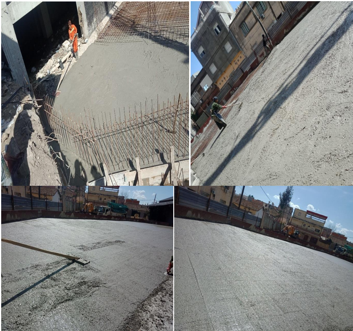
Figure I-21: Surfaçage de la dalle
