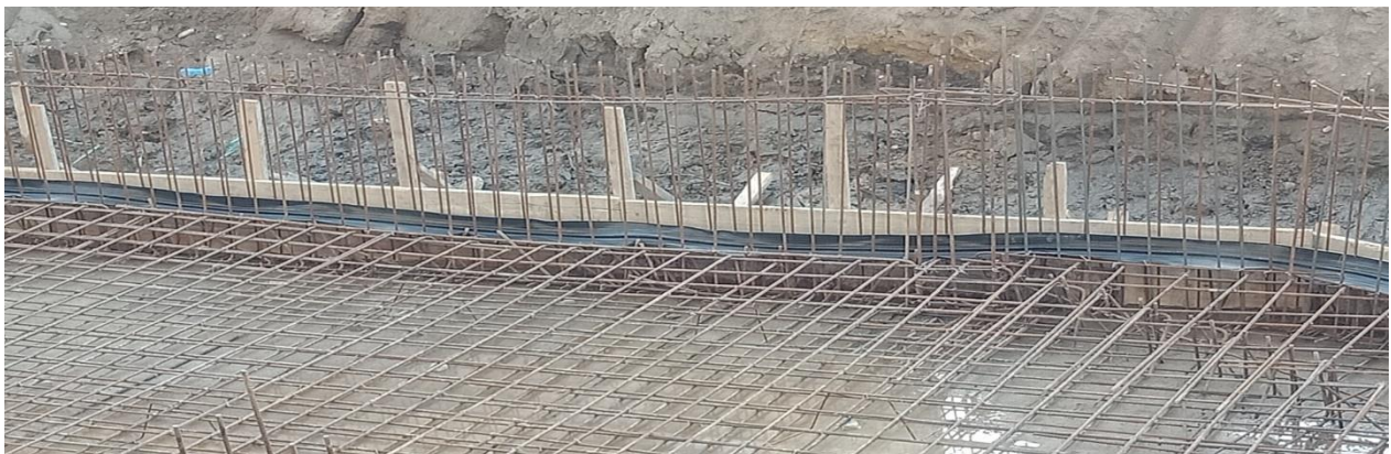
Figure I-18: Mise en place de joint Water stop
