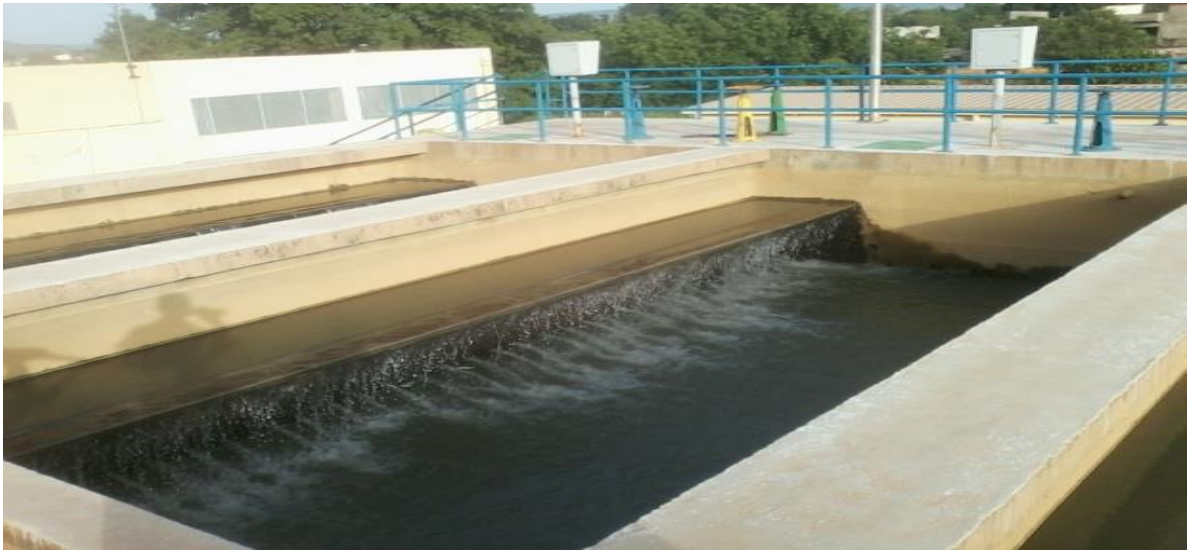
Figure III – 4 : Filtre aquazur V
