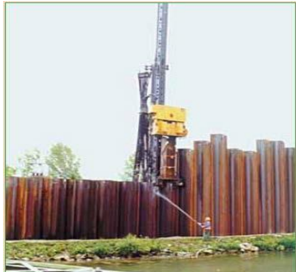
Figure I.20 Chantier de battage.[14]
