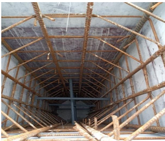
Figure I- 22-23 : ferrailages poteaux
