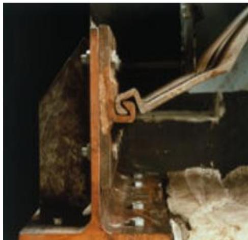
**Figure 2.19 Raccordement Omega**
