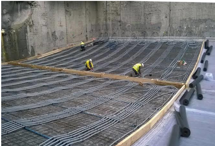
Figure II.20 : armatures de radier
