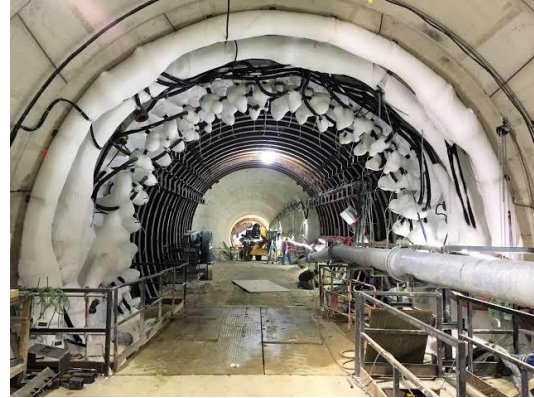
Figure II.9 : machine d'injection de consolidation Figure II.10 : congélation
