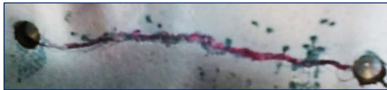
Fig. 4.13. Limiting the crack through holes
