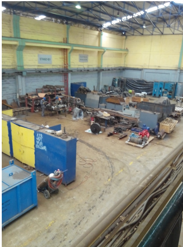
Figure II.7 L'atelier de maintenance
