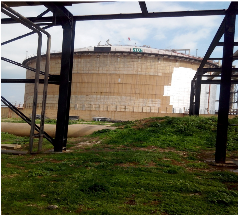
Figure III.8 Le Bac de stockage d'ammoniac de Ferial
