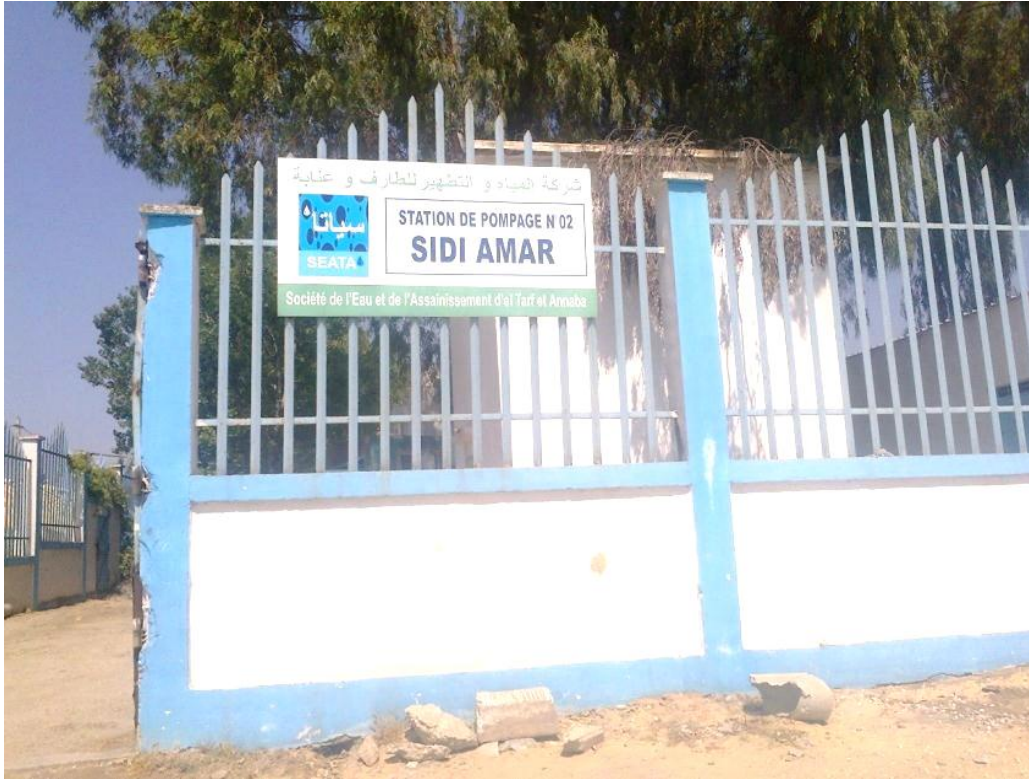
Figure IV.8 : Station de pompage existante SP2
