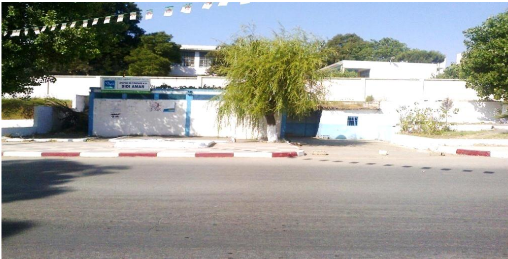
Figure IV.1: Station de pompage existante SP1
