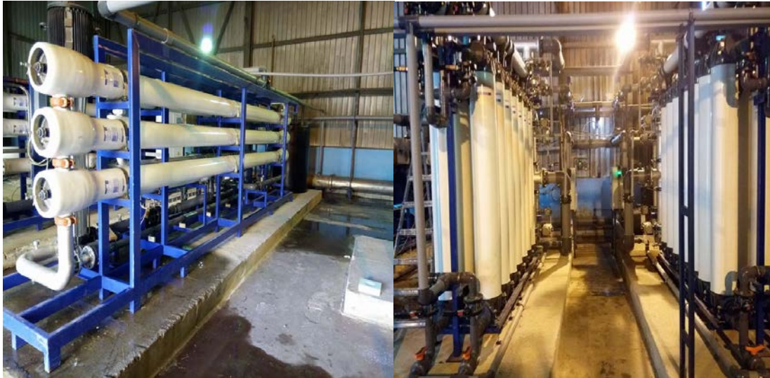
Fig.I.13: Installation d'osmose inverse.
