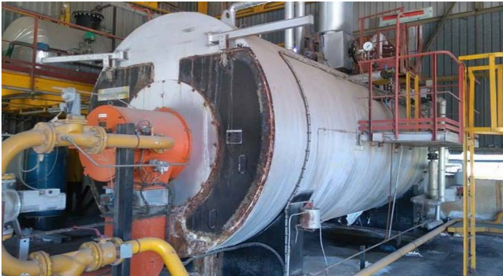
Figure I.17: Chaudière N°1 de la zone Est.
