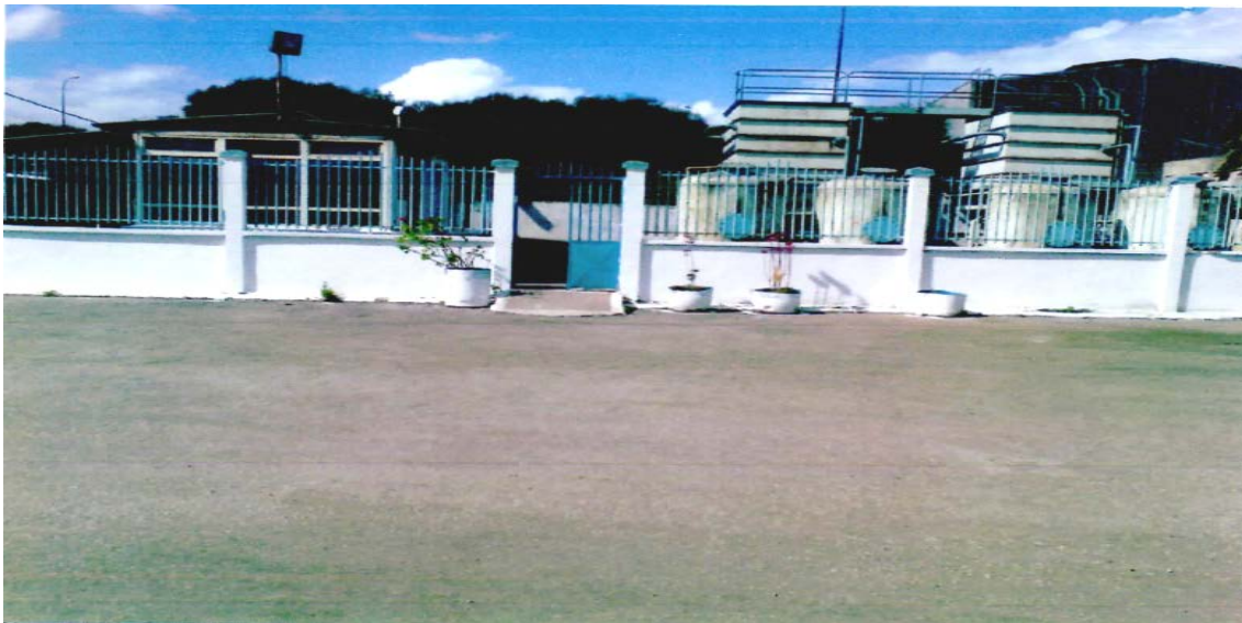
FigureI.18: Station de l'eau potable.
