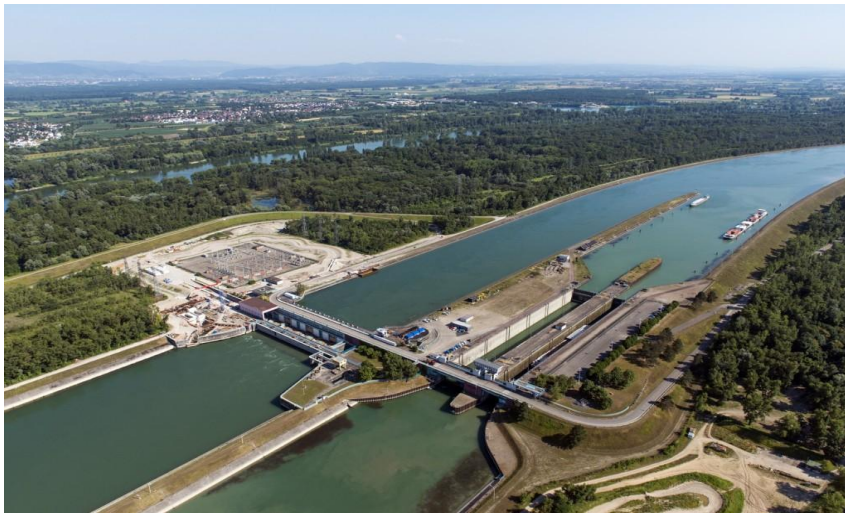
Figure (I-4) : centrale hydraulique
