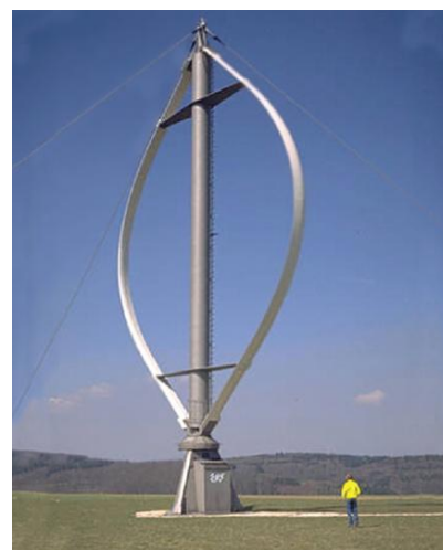
Figure I.6 : rotor de Darrieus
