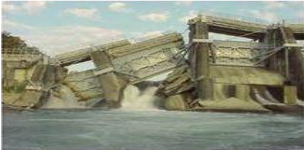
Figure 1.5 : Rupture de barrage Shihkang (Taiwan). {2}
