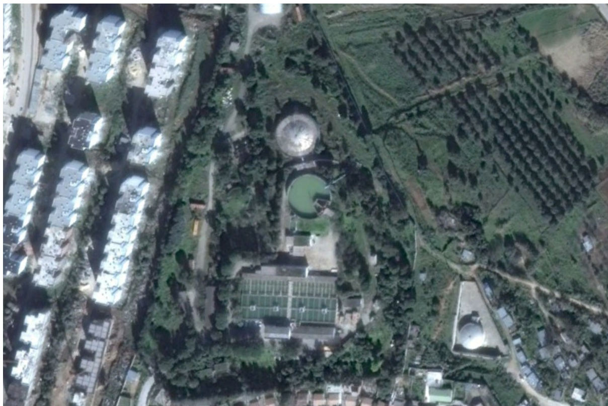
Figure.35: Station de traitement de chaiba (photo GOOGLE EARTH).
