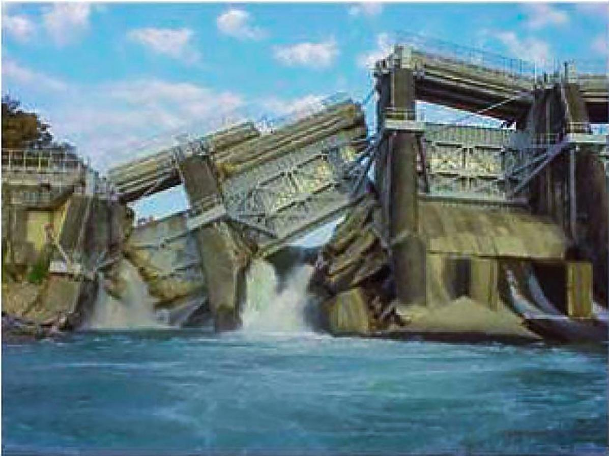
**Figure1.12:** rupture de barrage Shihkang (Taiwan) [53]
